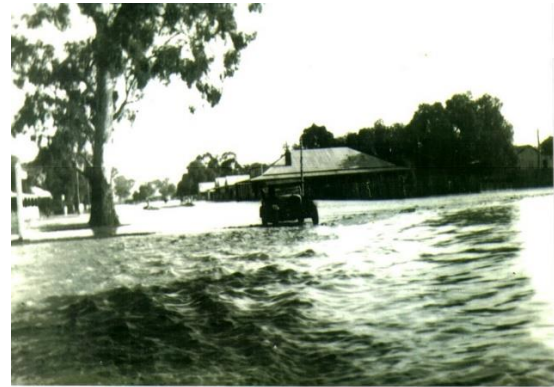
Photo 4-10: 1930's flooding on the corner of Mary Gilmore Way and Grenfell Street
