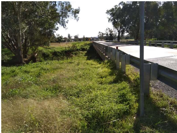
Photo 4-1: Mary Gilmore Way Bridge over Burrangong Creek
