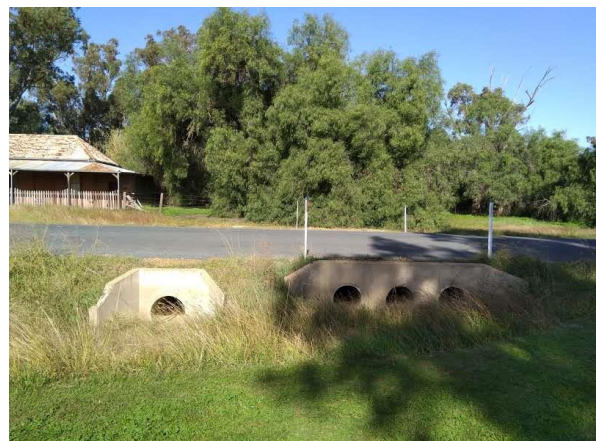
Photo 4-4: Culverts under Grenfell Street, north of Caldwell Street
