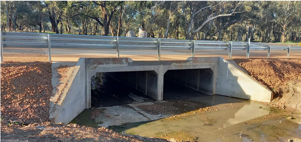
Photo: Adelargo Road culvert replacement project with guardrails
