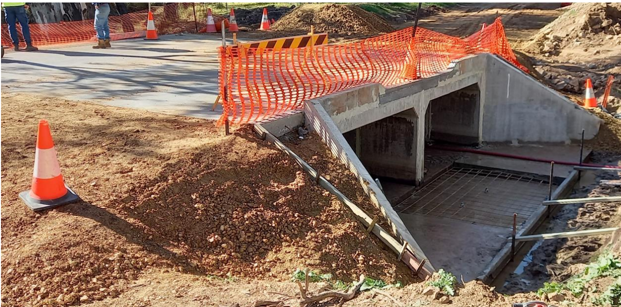
Photo: Adelargo Road culvert under construction
