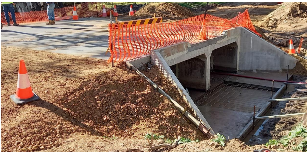
Photo: Adelargo Road culvert under construction
