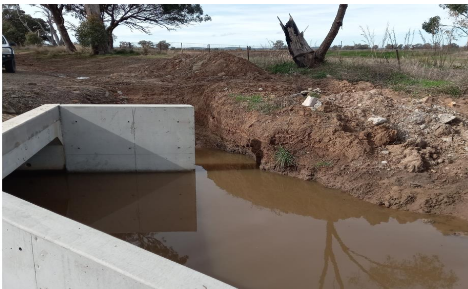
Photo : Back Piney Range Road - Culvert Site
