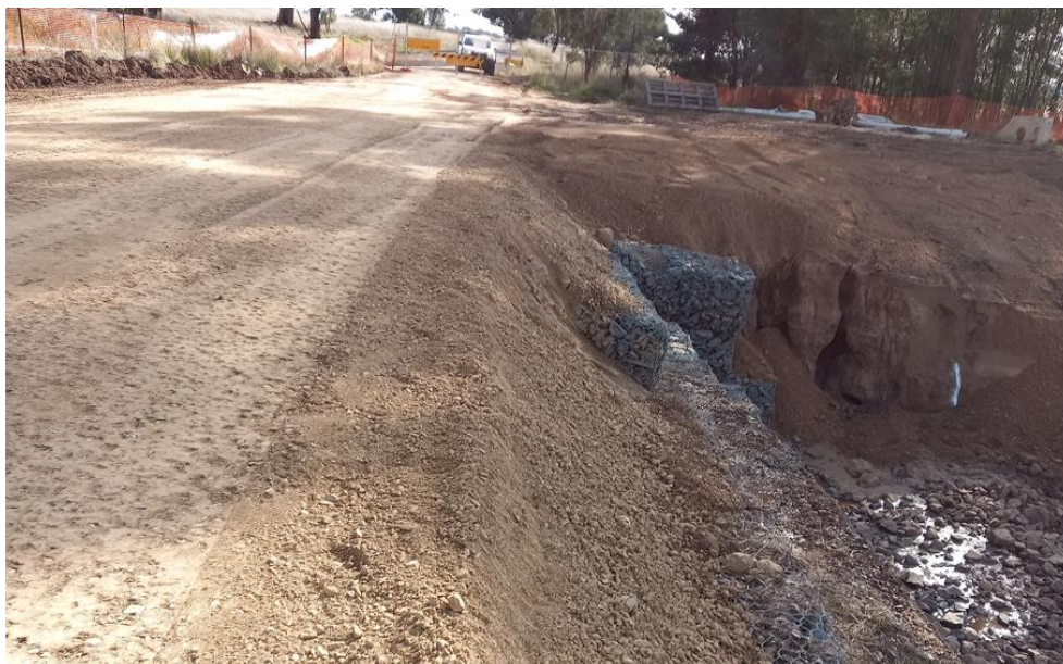
Photo : New Forbes Road – Culvert Replacement Site
