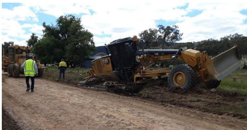
Emergency work that was completed on Kangaroo Road from the previous storm event again suffered damage at two (2) culverts where the road base was washed away. Repairs were again completed to enable farmers access to/from their properties. There is still more emergency work to be completed as time and resources permits.
