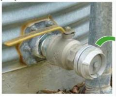
Reason: Requirement of 'Planning for Bush Fire Protection 2006' guidelines for adequate water supply for fire fighting.
