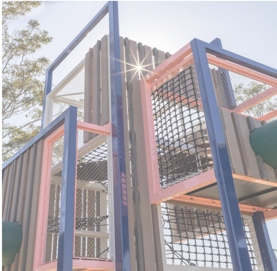
13 Lizard Lookout provides a custom made play element within a sculptural tree trunk, which references the habitat of the Goanna. An internal ramp offers an exciting journey for all to the lookout, a net for lying and looking up to the sky, and a dignity slide down to repeat it again and again! Ladders and other hand-holds provide alternate play routes up the tree trunk.
