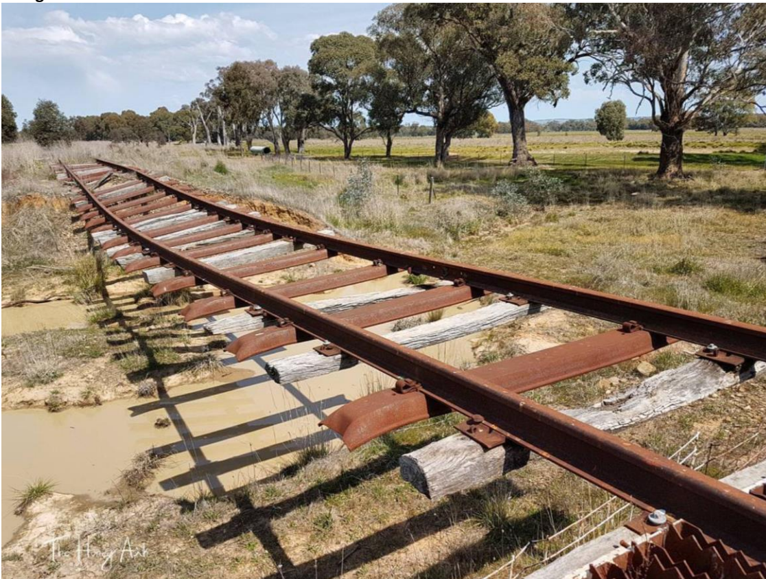
Figure 10.4 Images of the condition of the railway line – with parts of the line being flood damaged and other parts overgrown.
