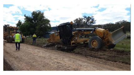
Emergency work that was completed on Kangarooby Road from the previous storm event again suffered damage at two (2) culverts where the road base was washed away. Repairs were again completed to enable farmers access to/from their properties. There is still more emergency work to be completed as time and resources permits.
