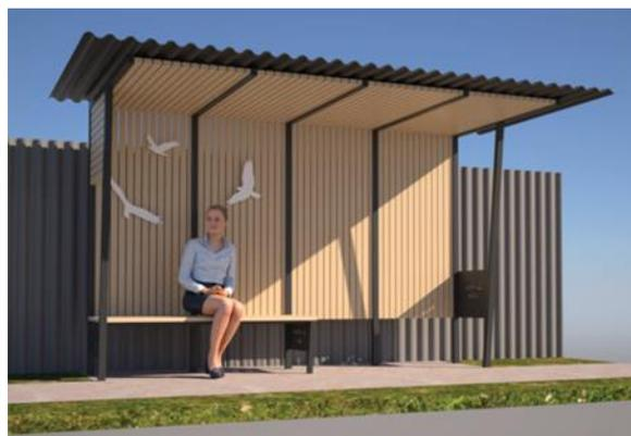
The Bus Shelter has been designed to the restrictive width of the footpath along Forbes St, hence the cantilever design.
